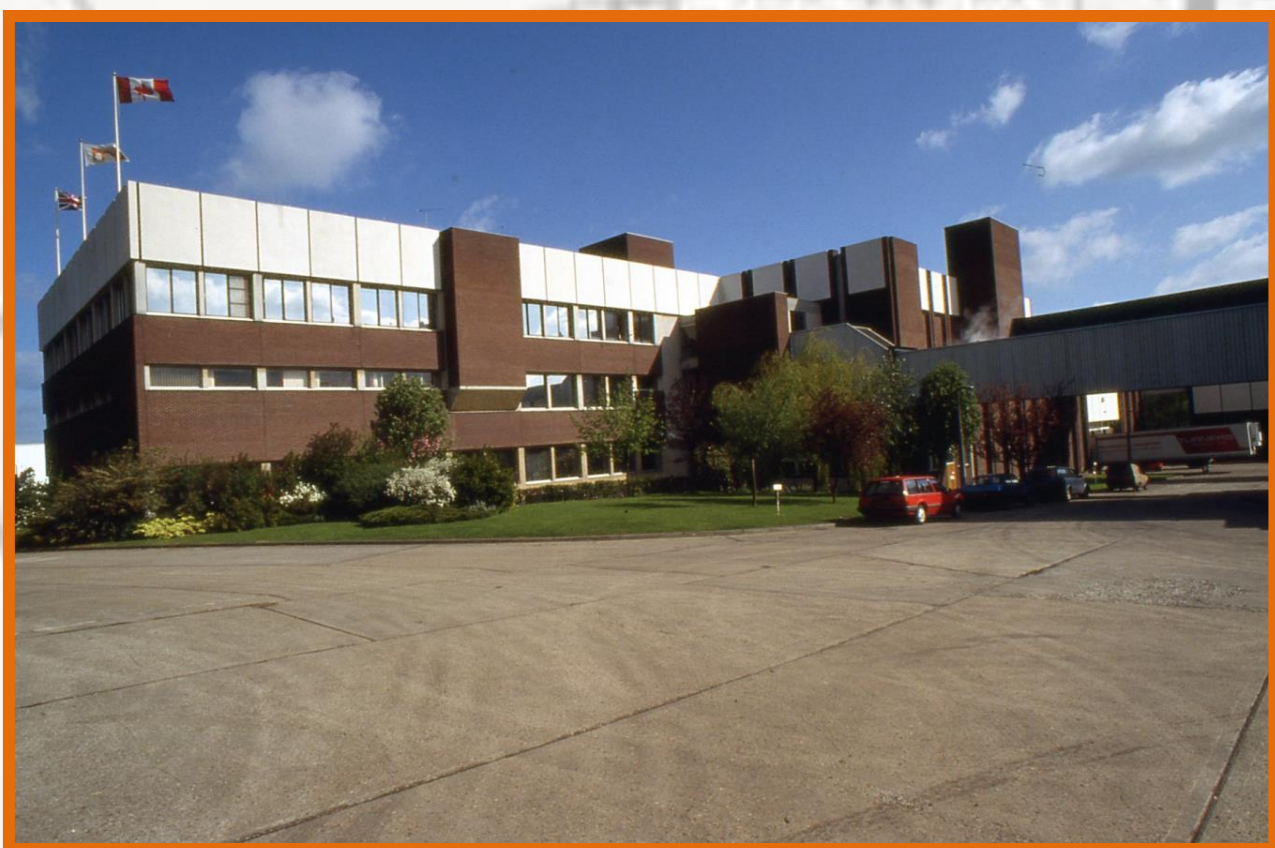
Office block & factory from the main gate
