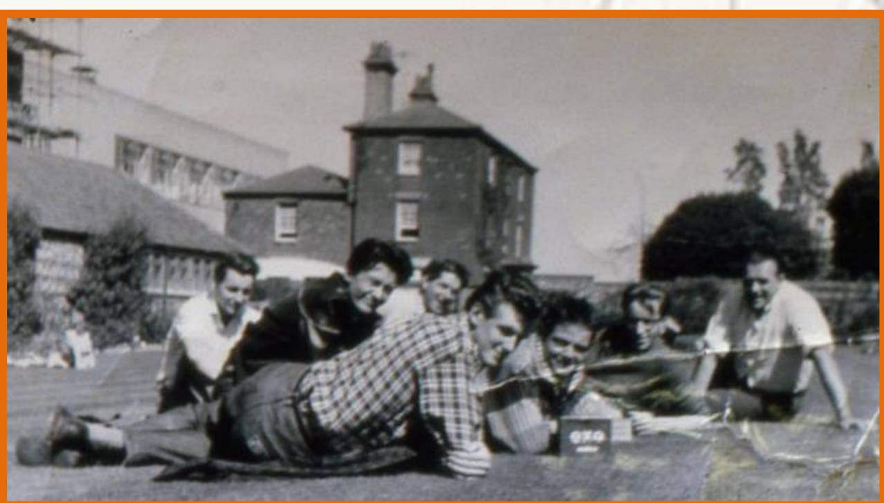
Break on Blunts Hall lawn c1961 with Roy Taylor & Sooty Thake (right). 2nd phase of plant under construction.
